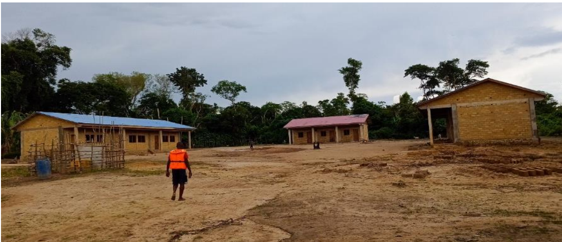
Figure 4.1. School construction in Inunu.
